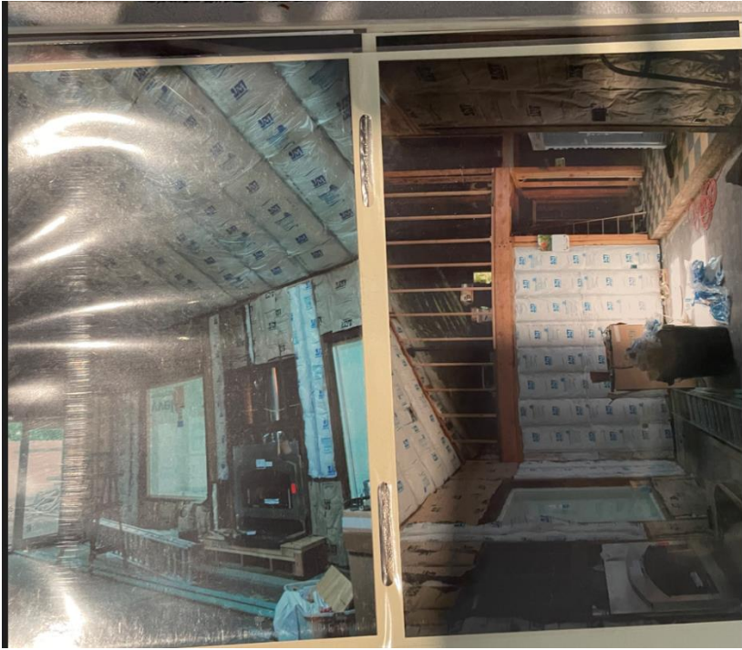
Image showing removal of program insulation during remodel event for site WI_11.
